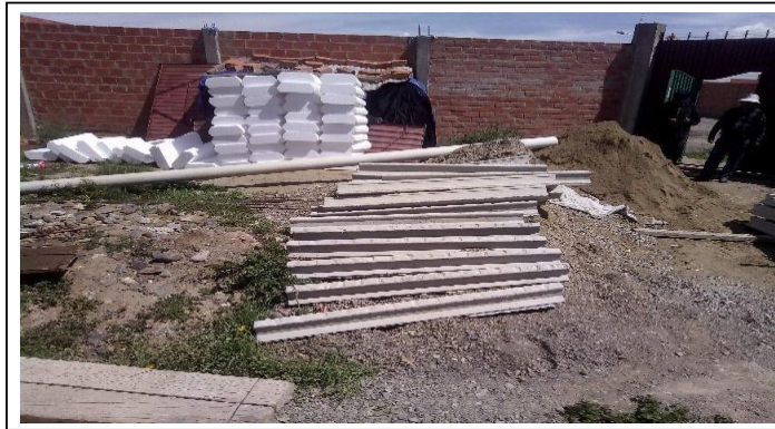
IMAGEN 1: CEMENTO PORTLAND (50KG), PLASTOFORM 100X40X16
