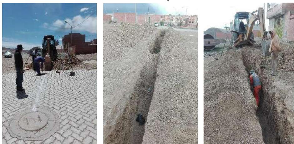
**IMAGEN 2: TENDIDO DE TUBERIA, RELLENO Y COMPACTADO**
