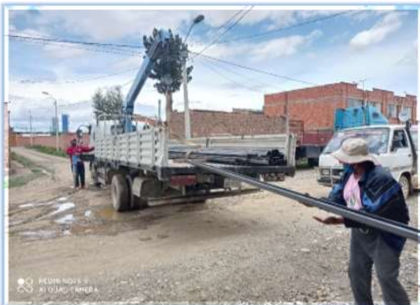
Perfil costanera 100x50x15x2mm (barra=6m)
